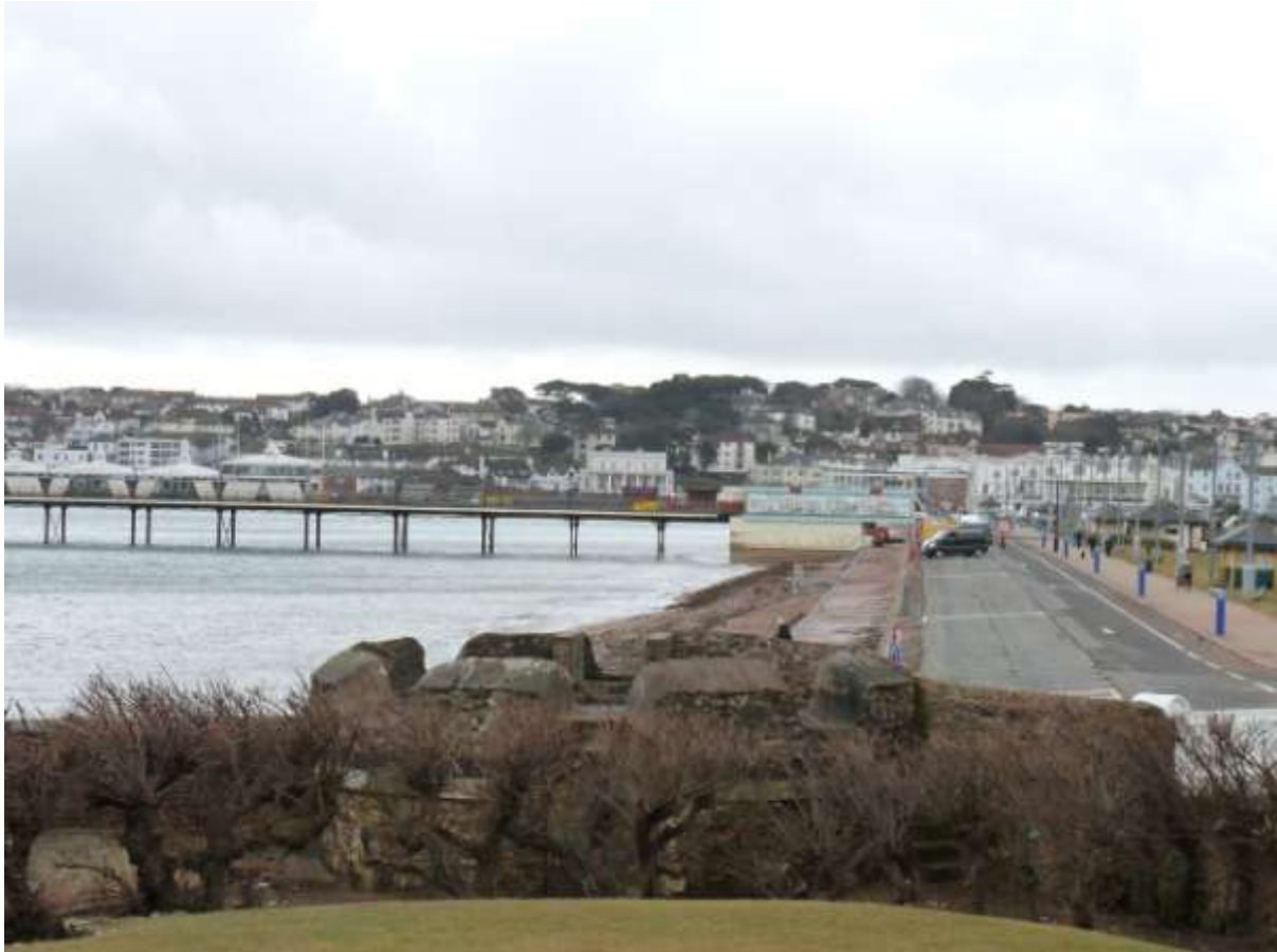
Figure 15. The remains of one of the flagstaff towers, once a prominent feature it stands half-buried in the undergrowth. Photograph by Diane James © 2013.
